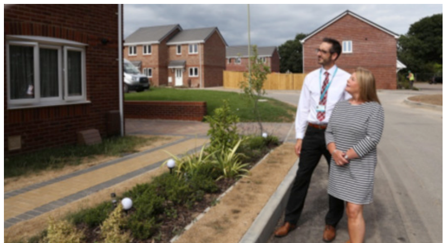
New build Council properties in Lymington, 2018
